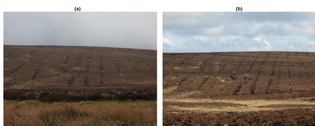
Figure 4. Drainage ditches before (a) and after (b) blocking on a blanket bog in North Wales: the ditches run down the slope and individual dams can be seen crossing the ditches (photos: Chris Evans).
