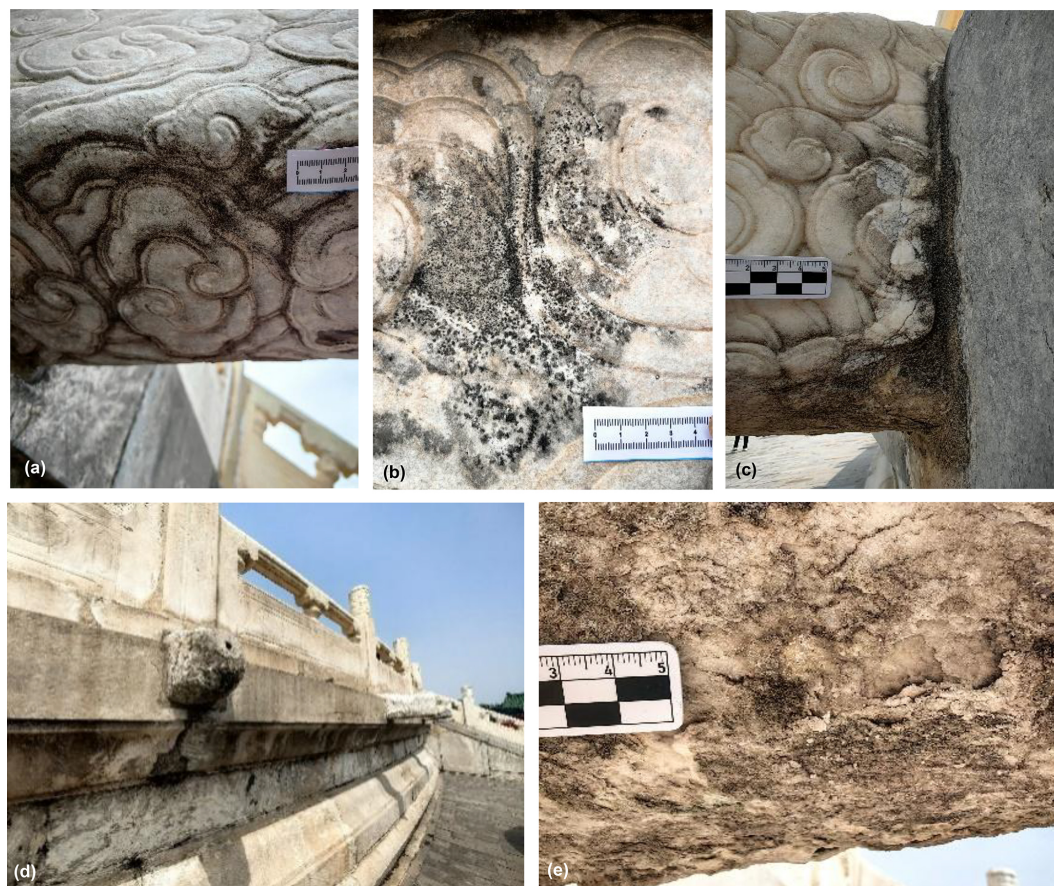
Figure 23. Bioweathering process of the Cloud Chi Head on the Hall of Prayer for Good Harvests in the Temple of Heaven, Beijing, China: (a) The organisms gather and grow in the low-lying areas of the Cloud Chi Head ornamentation; (b) The organisms gather and grow in the low-lying areas of the Cloud Chi Head ornamentation; (c) The surface of the Cloud Chi Head is flaking off in patches; (d) The Cloud Chi Heads have even weathered away completely; (e) A loose, powdery layer has formed on the surface of the Cloud Chi Heads, with a large amount of cyanobacteria growing inside.
