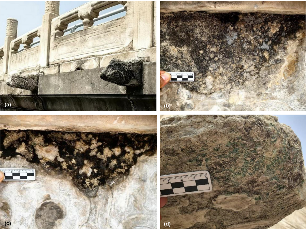
Figure 14. Field photo of biomes on the south facing marble surface of the altar of Prayer for Good Harvest in the Temple of Heaven, Beijing, China: (a) Some carved decorations have been completely destroyed; (b) Gray-white, Gray-black; (c) Black leathery; (d) Green powdery layer.
