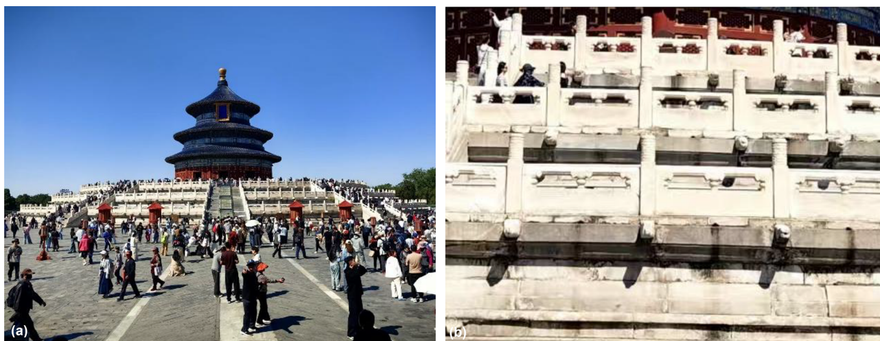
Figure 1. The hall of Prayer for Good Harvests in the Temple of Heaven, Beijing, China, and the distribution of black biofilm on its marble surface: (a) The Hall of Prayer for Good Harvests has a base consisting of three tiers of marble platforms; (b) The surface of marble platforms is covered with black biofilm, which is distributed according to the intensity of rainfall. In areas with low rainfall intensity, the biofilm is not noticeable. In areas with high rainfall intensity (such as channels, water convergence points, and Chi Heads), there is a significant distribution of black biofilm.
