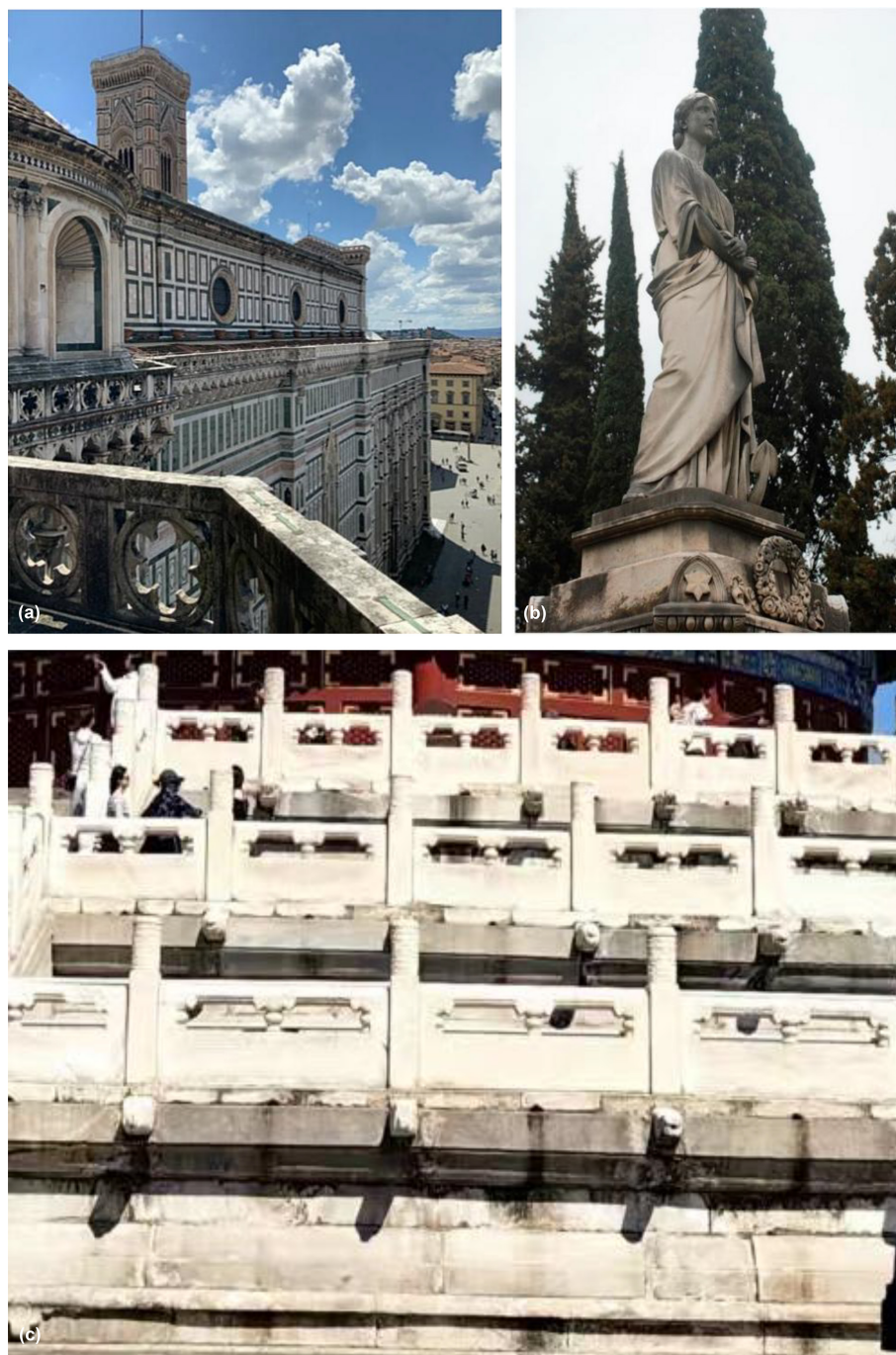
Figure 24. Comparison of Black Biofilm Growth on Marble Relics in Florence and Beijing: (a) Cathedral of Santa Maria del Fiore in Florence (façade completed in 1887, 138 years old, using white, green, and pink marble), with a large area covered by black biofilm (Santo et al., 2023); (b) Speranza statue in Florence (built in 1863, 158 years old, using white marble), with a large area covered by black biofilm (Mascalchi et al., 2018); (c) The Hall of Prayer for Good Harvests at the Temple of Heaven in Beijing (built in 1420, 605 years old, using white and bluish-white marble), with a small area covered by black biofilm, mainly distributed in areas with high runoff from sudden rain.
