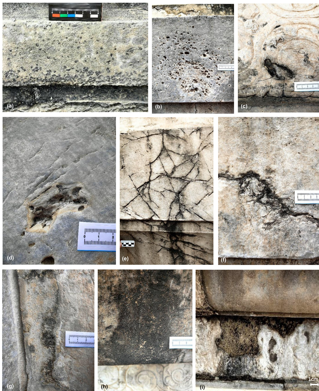
Figure 22. Bioweathering forms on the marble surface of the Hall of Prayer for Good Harvests in the Temple of Heaven, Beijing, China: (a) biological community point distribution; (b) Solution pores and solution cavities; (c) Sinkhole; (d) Solution pit; (e) biological community linear distribution; (f) Solution marks and solution grooves; (g) Solution channel; (h) biological community areal distribution; (i) Spalling layer.
