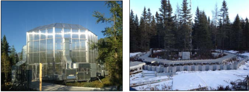
Figure S4: Left photograph is a completed SPRUCE warming enclosure, and the right photograph shows the subtending hydrologic corral that lies beneath each enclosure. The encircling and interlocked sheet piles extend through the peat to the ancient lake bed below, and effectively isolate the hydrology of the enclosure.
