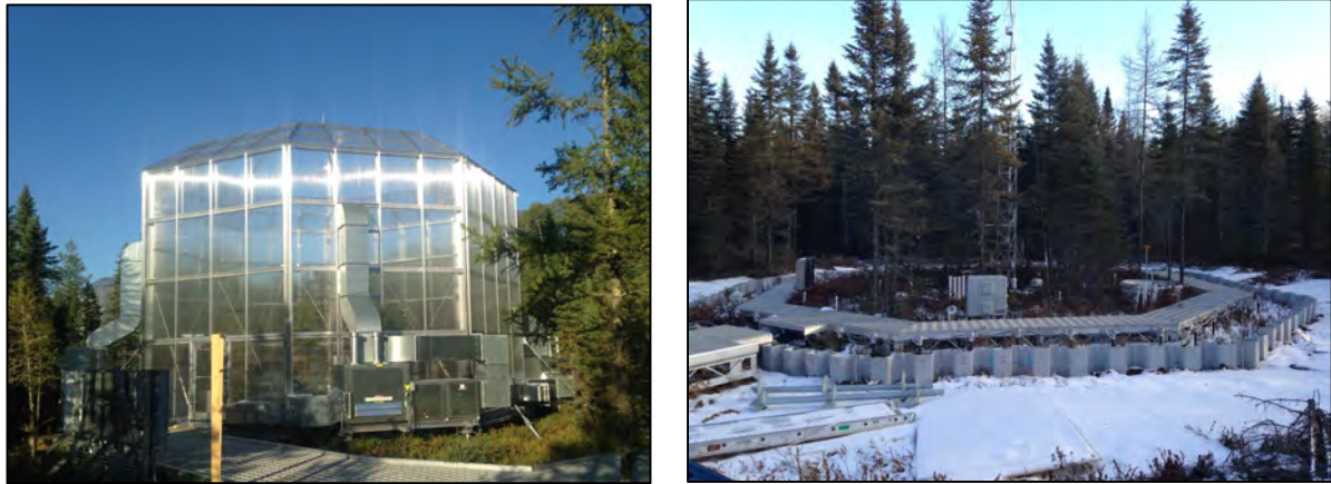
Figure S3: Left photograph is a completed SPRUCE warming enclosure, and the right photograph shows the subtending hydrologic corral that lies beneath each enclosure. The encircling and interlocked sheet piles extend through the peat to the ancient lake bed below, and effectively isolate the hydrology of the enclosure.
