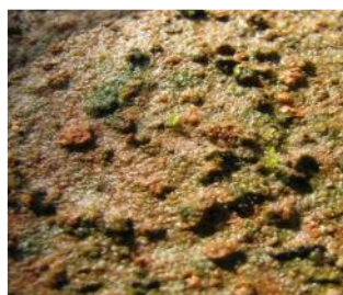
Type 1 Crust formation - increased chlorophyll content as cyanobacteria grow and form a smooth surface crust
