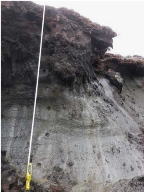
Figure S3: Drained thermokarst lake basin exposure BAL16-B3. Photo by J. Strauss, August 2016.
