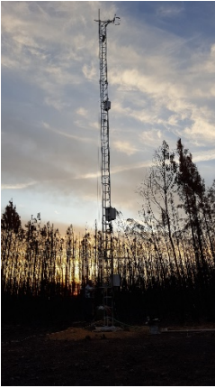
Figure 4. The 12 m slim tower with the eddy-covariance system immediately after its installation (Photograph: J. Jacob Keizer, 22 September 2017).
