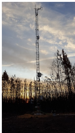
110 Figure 3. The 12 m slim tower with the eddy-covariance system immediately after its installation (Photograph: J. Jacob Keizer, 22 September 2017)
