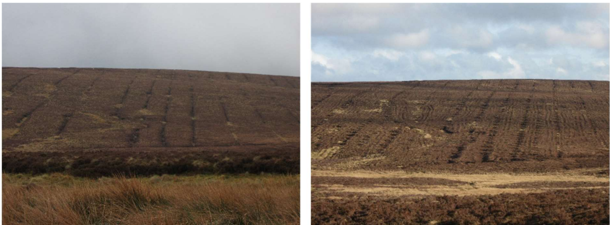
866 Figure 4: Drainage ditches before (left) and after (right) blocking on a blanket bog in North Wales, the ditches run down 867 the slope and individual dams can be seen crossing the ditches (Photos: Chris Evans).
